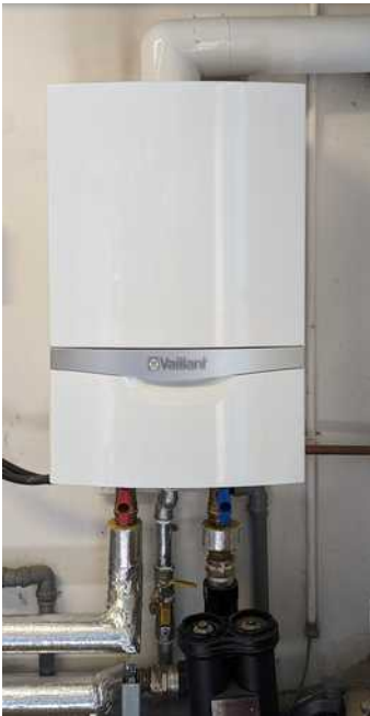
60 kW replacement boiler installed in child care building at 134 Stewartstown Road – September 2021
